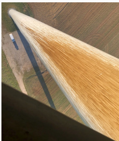
Oil leak due to crack in yaw tank in France without ground pollution:
